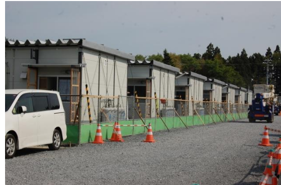
Temporary housing in Rikuzentakata City
