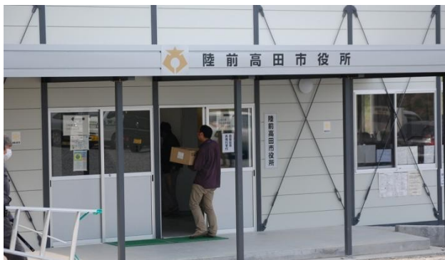
The temporary town office in Rikuzentakata City
