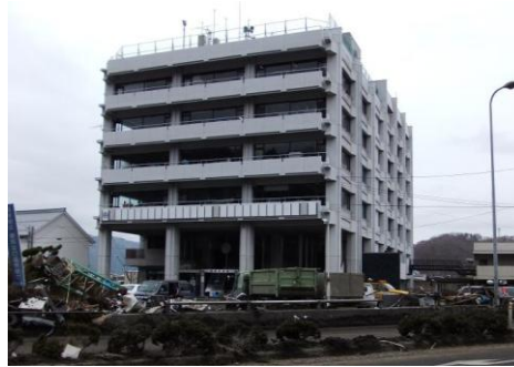
The Miyako City Hall. The first and second floors were damaged. The electricity and the Internet were out.
